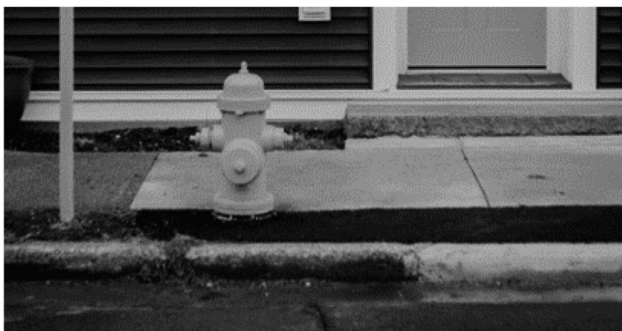
Newly painted hydrant on Little River Road, Flamborough. The project has taken two years to complete
