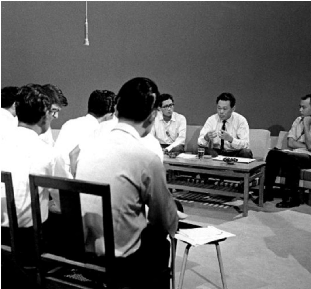
Meeting the press on the morning of Singapore's separation from Malaysia, 9 August 1965.
