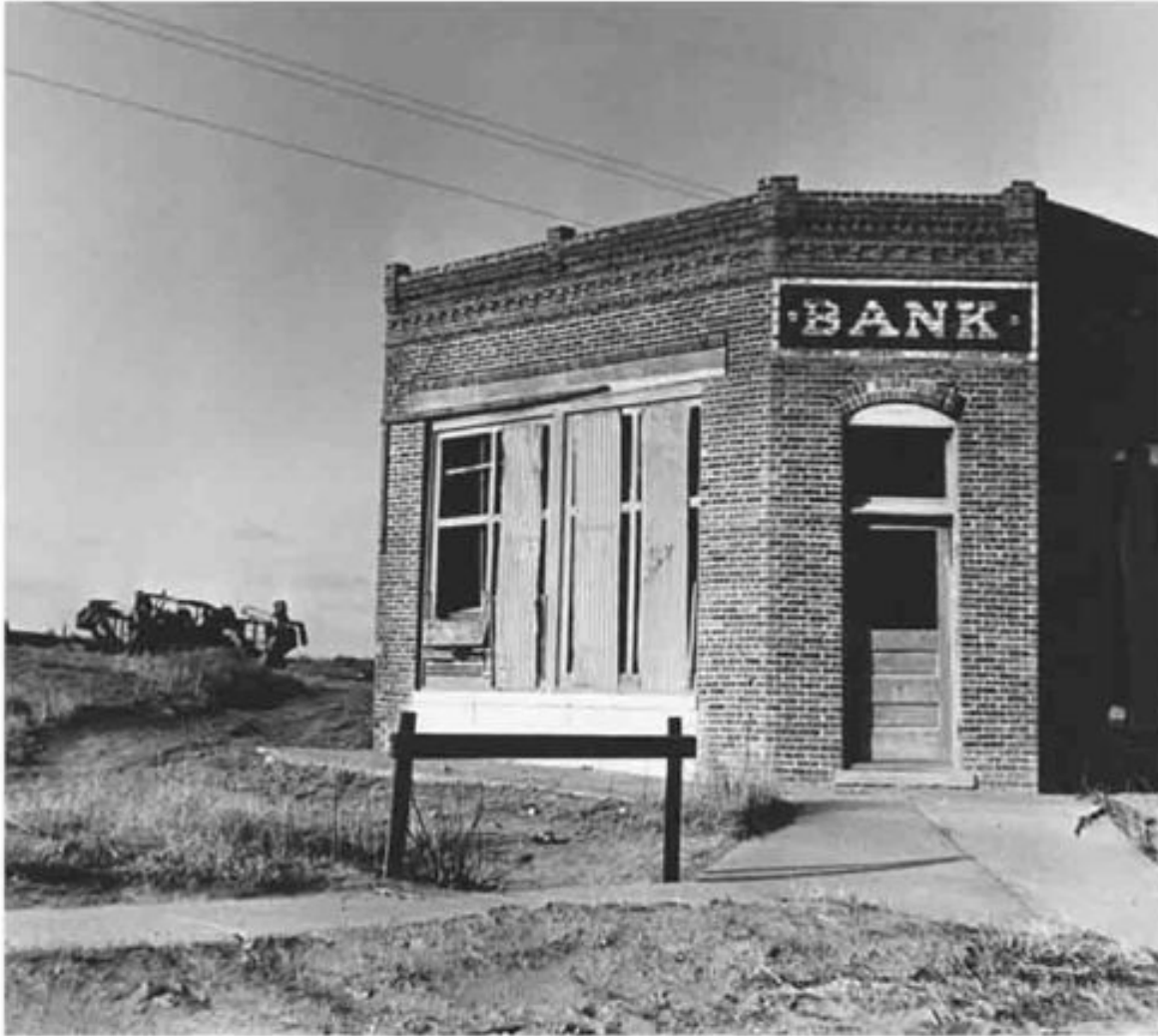
Failed bank, Kansas, 1936
