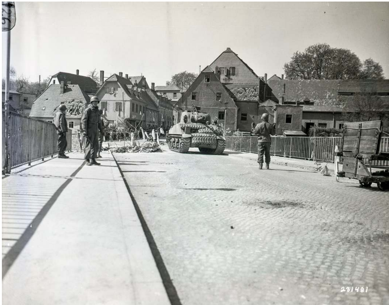
American troops cross Colditz bridge, with visible damage from the failed German attempt to destroy it.
