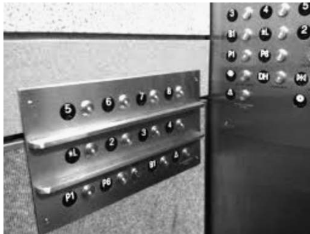
Horizontal and vertical elevator buttons inside an elevator at the U.C.S.F. Ambulatory Care Center, 400 Parnassus Avenue, San Francisco.
