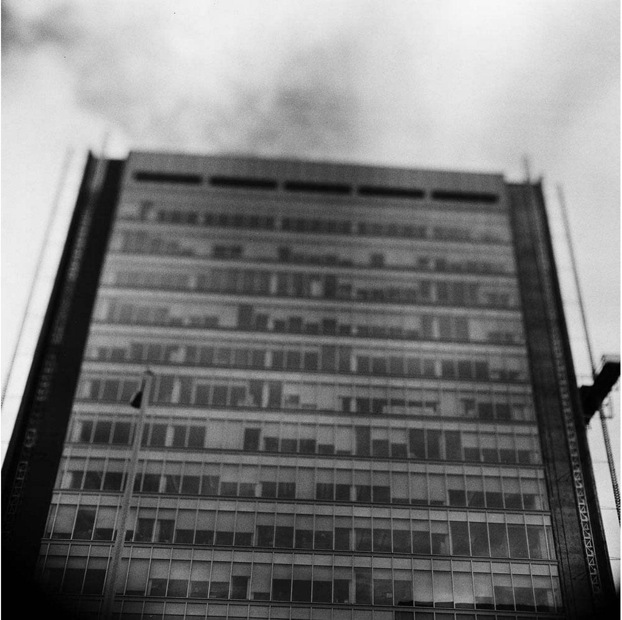
Poff Federal Building, Roanoke, Virginia
