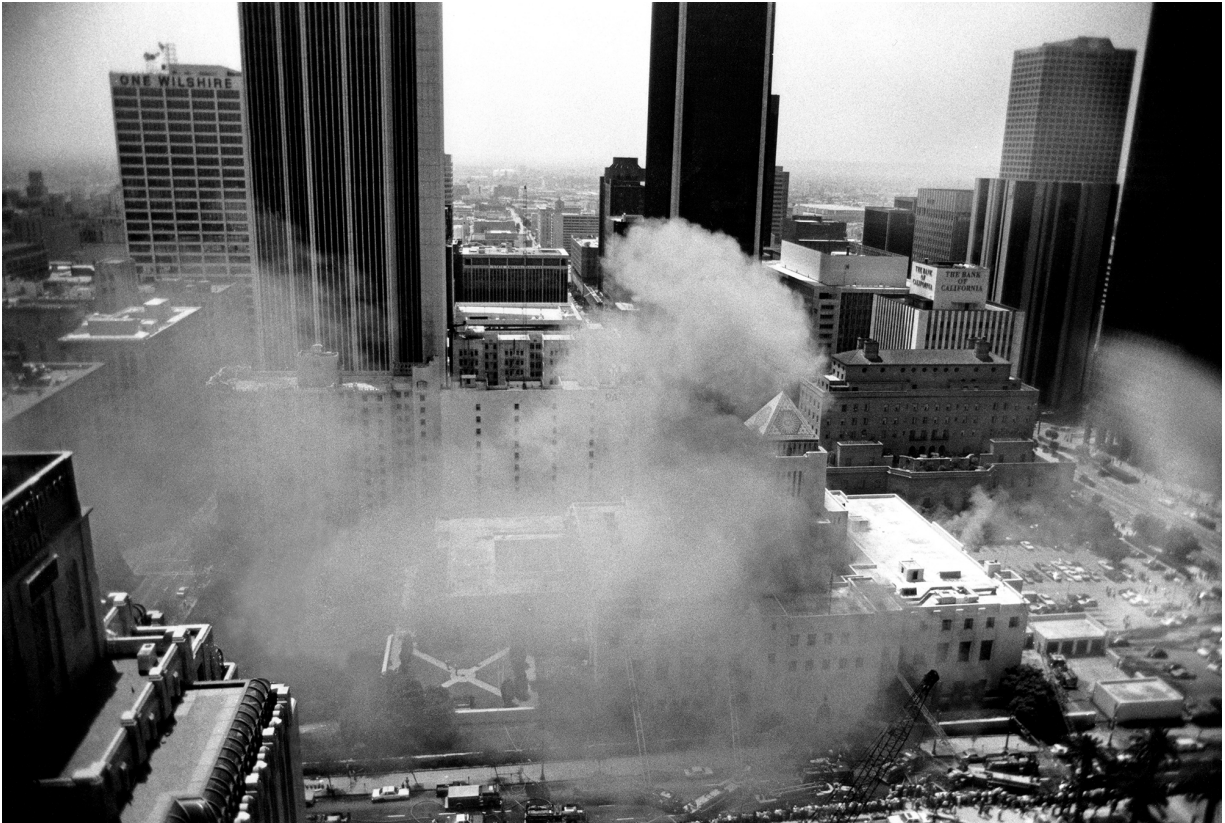
The fire as seen from Fifth Street
