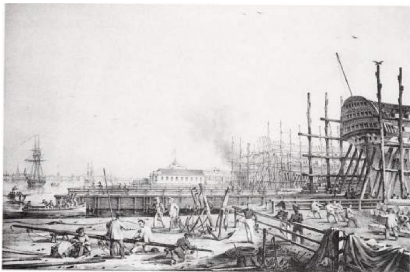
8. Admiralty Wharf: the construction of the Russian navy
