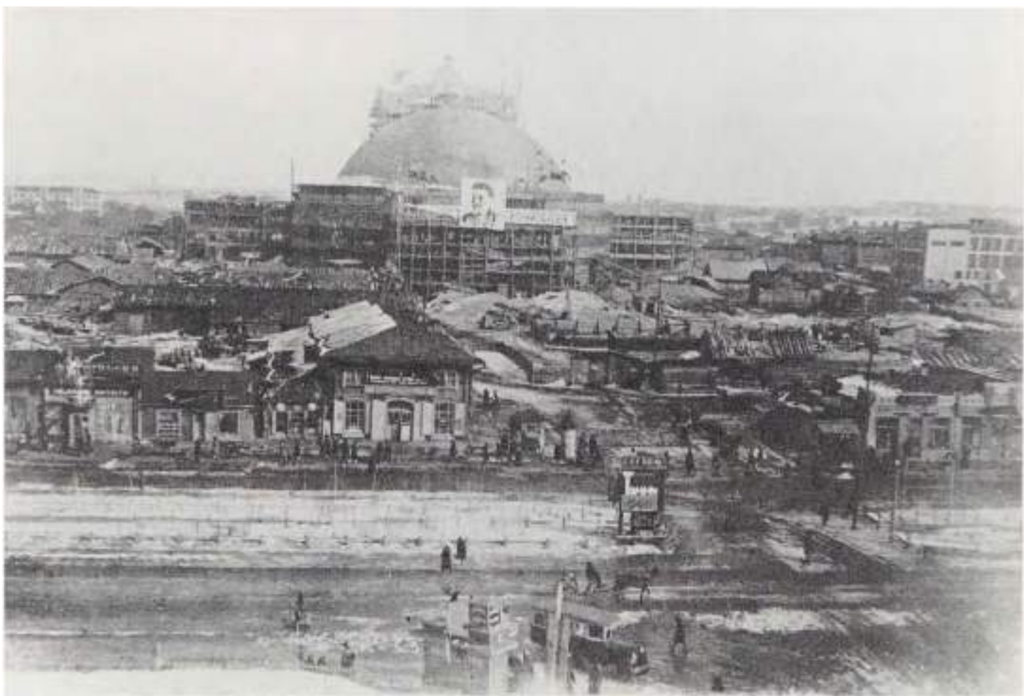
29. Construction of the opera house. Novosibirsk, late 1930s
