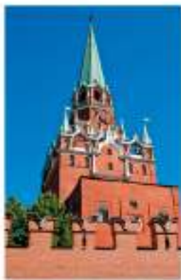
The seven-storey Trinity Tower, the tallest tower in the Kremlin
