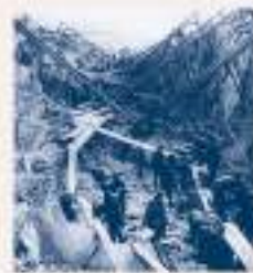
Prisoners at the construction site of the White Sea Canal
