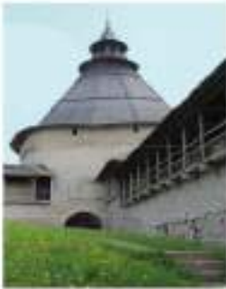
Pokrovskaya Tower, a part of Pskov's outer ring of fortifications
