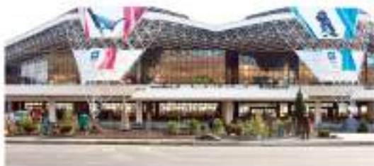
The three-level air terminal complex at Sochi International Airport
