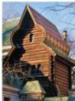
Ornate roof of the wooden house designed by Viktor Vasnetsov
