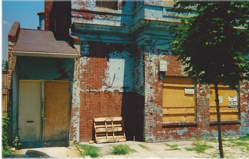
THE ENTRANCE TO THE FAMILY FLAT OVER THE GROCERY STORE, CA. 1943.
