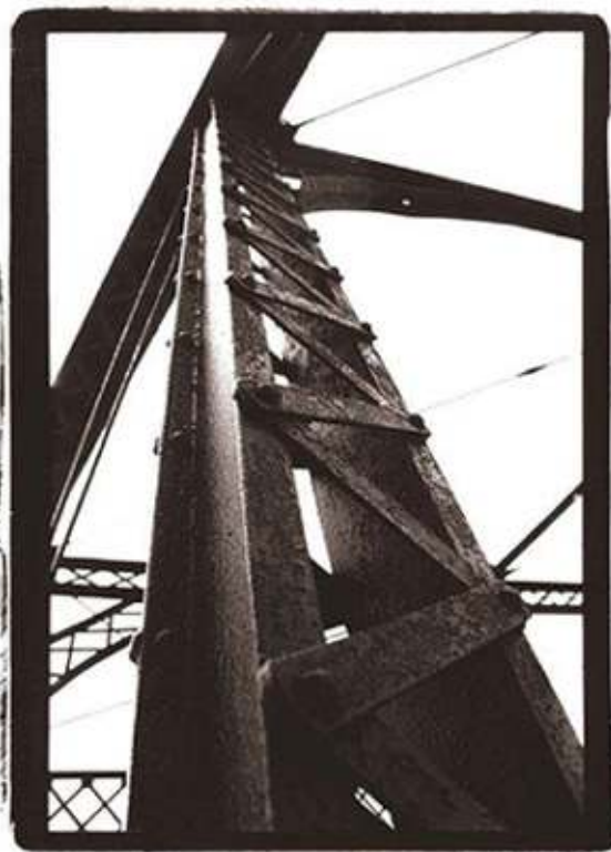
Washington Street Bridge. 1999.
