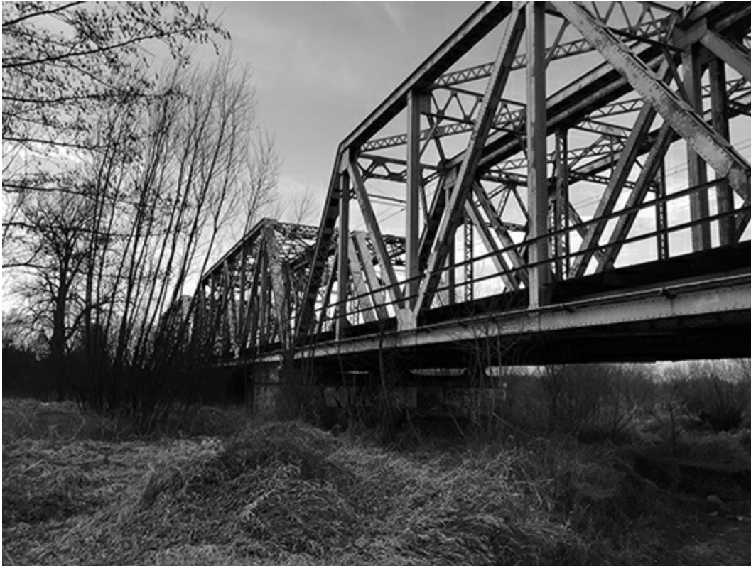
Bridge over the Soła River.
