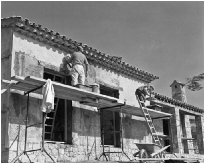
Building La Pitchoune
