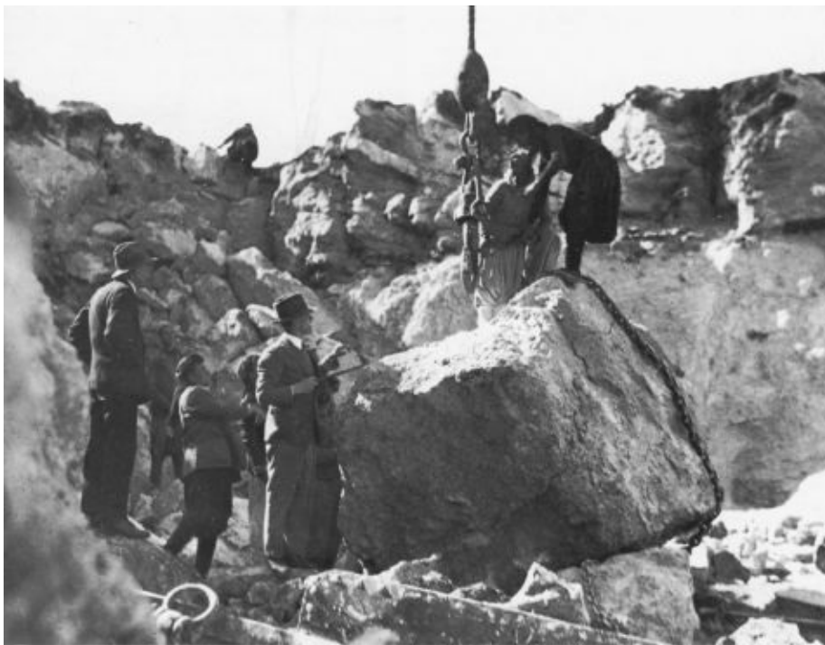
Figure 4 The Atlit stone quarries, where Arabs and Jews were jointly employed
