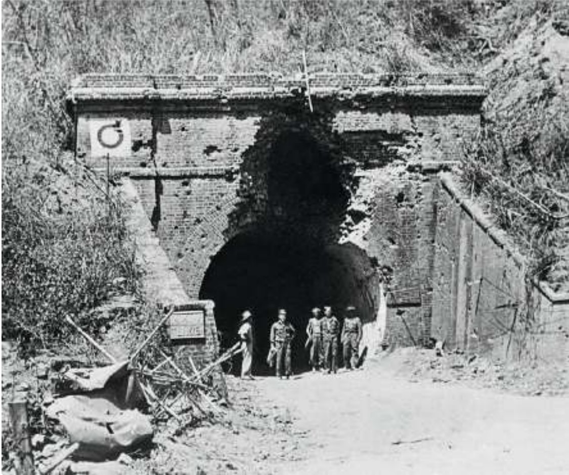
Entrance to one of the heavily defended tunnels on the Maungdaw-Buthidaung road that we captured from the Japanese 55th Division.
