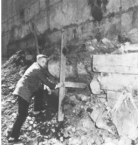
At age twelve, inspecting the foundation for a six-story building in Queens, New York.
