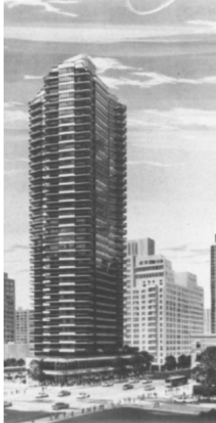
Model of Trump Plaza, a 175-unit residential tower located near Bloomingdale's at 61st Street and Third Avenue on New York's Upper East Side.
