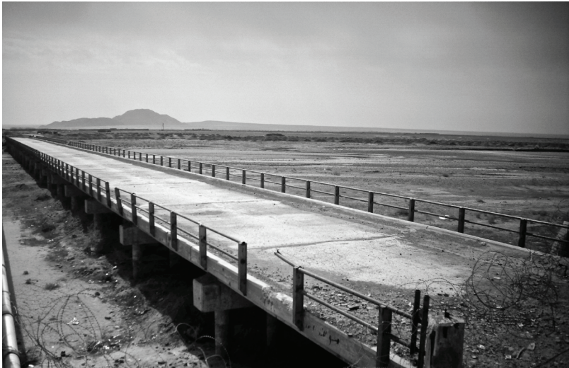
Arghestan Bridge, Kandahar province
