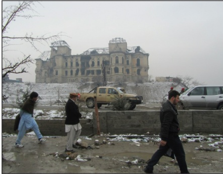
Darul Aman Palace, on the outskirts of Kabul, was constructed during the reign of King Amanullah Khan. Though its name means “abode of peace,” it was virtually destroyed during battles among rival mujahideen factions in the early 1990s.
