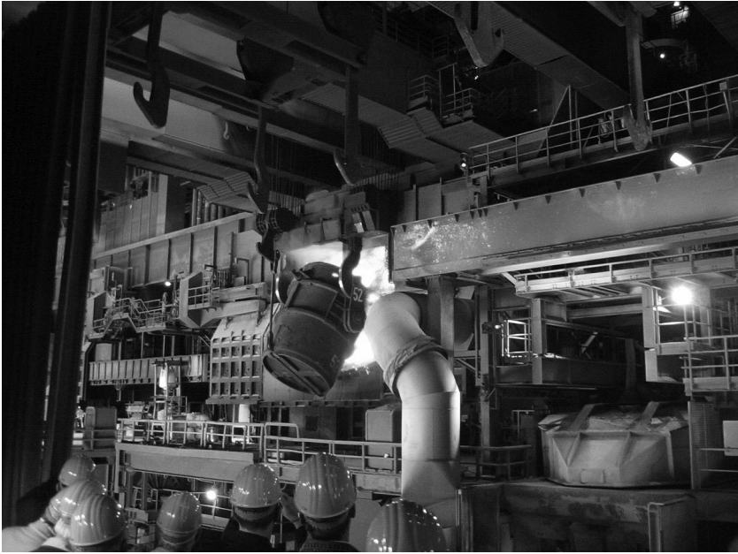
Figure 5.25 Basic oxygen furnaces, such as this one at ThyssenKrupp steelworks in Duisburg, dominate the global production of steel. Photo available at wikimedia.
