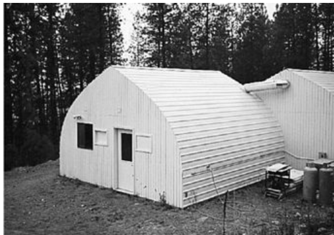
An insulated growing room constructed on the interior and exterior with weatherproof metal siding.
