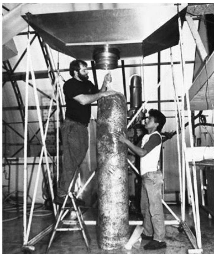
Once filled, the collar is released and the plastic is tied into a knot.
