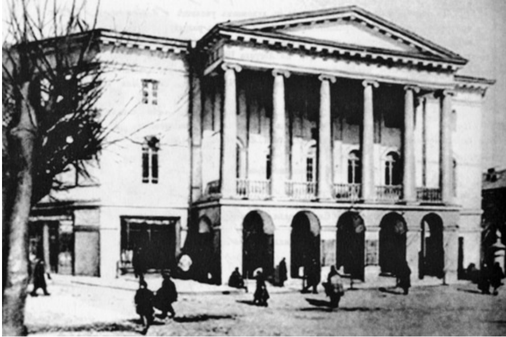
Neoclassical seminary building, dubbed the Stone Sack, where for a time Stalin lived as well as studied under a regimen of surveillance and snitching.
