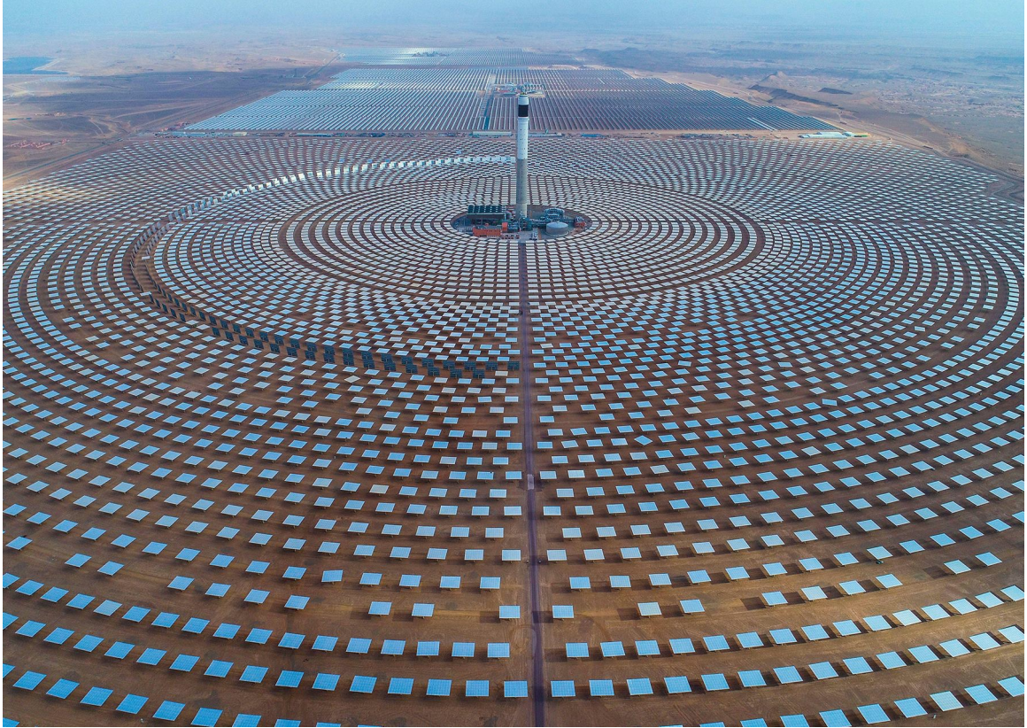
The Ouarzazate Solar Power Station in Morocco, the world's largest concentrated solar power plant, is built to supply electricity through the night using energy stored in molten salt. (© Xinhua/Alamy Live News)
