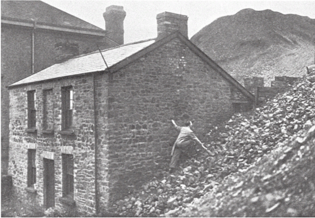
House near Swansea threatened by slag-heap
