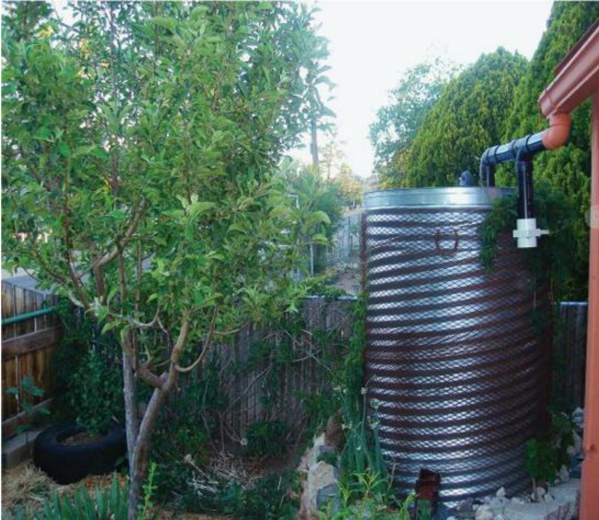
A 600-gallon rainwater tank made from galvanized metal culvert that gravity-irrigates a perennial front-yard garden in Prescott, Arizona, with trellising on the tank for vines. The warm microclimate created by the southwest exposure of the tank, which heats the water on sunny days and creates a warm microclimate, means that when there are late frosts the adjacent apple tree fruits only on the side facing the tank. PHOTO AND DESIGN BY ANDREW MILLISON OF MILLISON ECOLOGICAL DESIGN.
