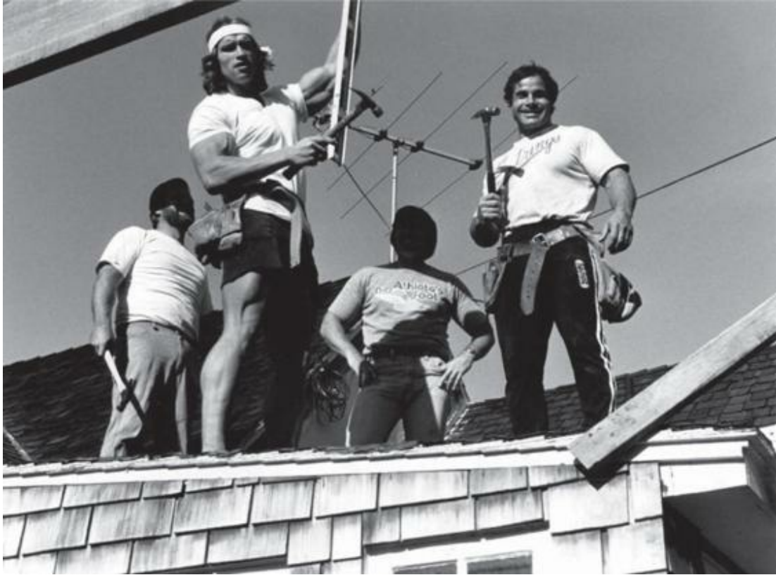
Franco Columbu and I billed ourselves as European experts in construction and hired other bodybuilders to help in our first business doing masonry and repairs. Art Zeller
