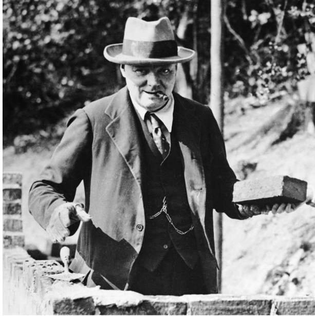
Winston Churchill, bricklayer, building a wall at Chartwell in 1928.
