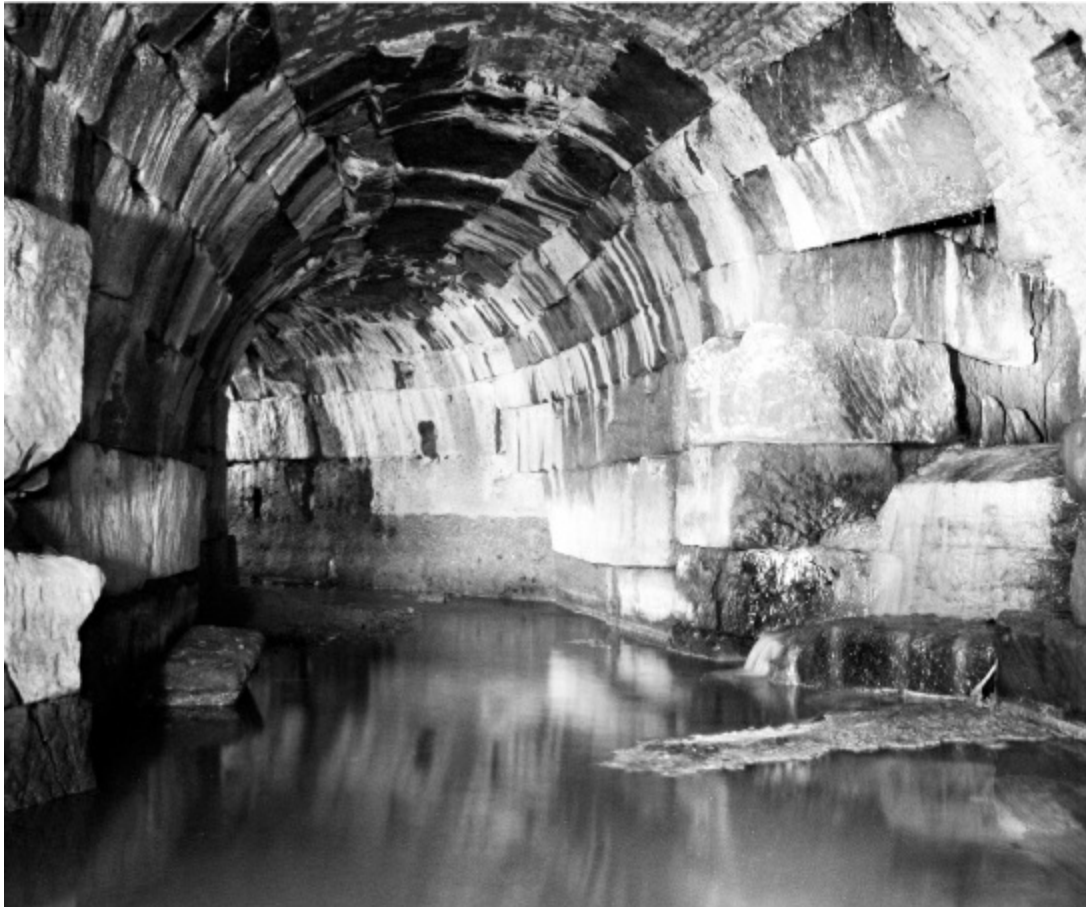
22. A surviving section of the underground Cloaca Maxima . The original drain can have been nothing like as grand as this later construction but this is the image that Roman writers had when they wrote of Tarquin’s building project. Some Romans boasted of taking boats and rowing along it.
