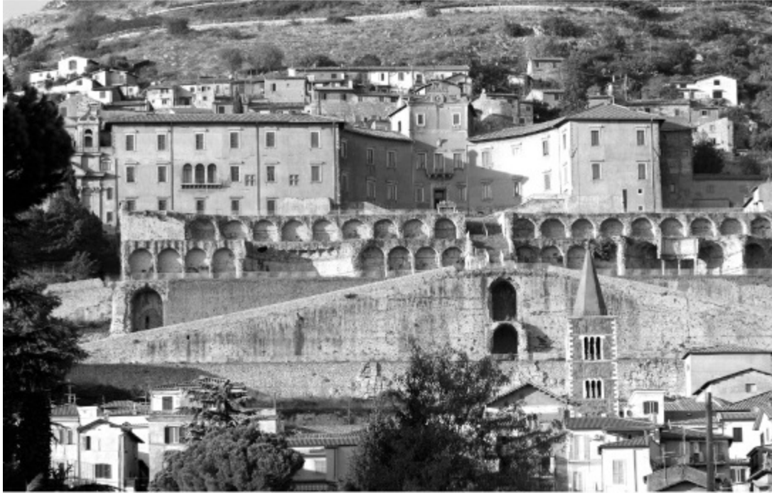
38. The huge architectural developments in late second-century BCE Praeneste were built into the later Renaissance palace, which still retains the basic shape of the ancient sanctuary. The lower ramps and terracing are still clearly visible.
